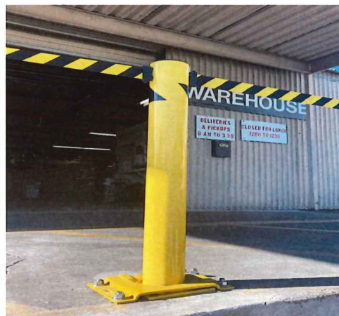
New removable bollards at the center of the dock area.
