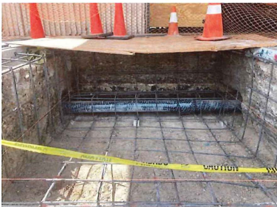
Demolition, excavation, and rebar installation for the foundation.
