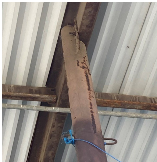
1. Hooks to be welded to existing columns to support the new shade coverings.
