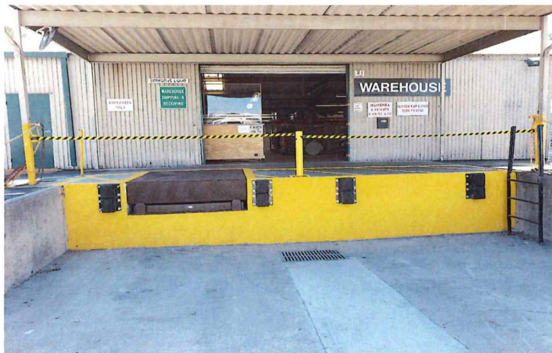
New dock leveler, bumpers, straps, and bollard installed at the Maintenance Warehouse.
