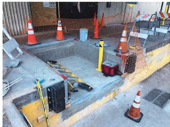
New concrete poured in preparation for the leveler installation.
