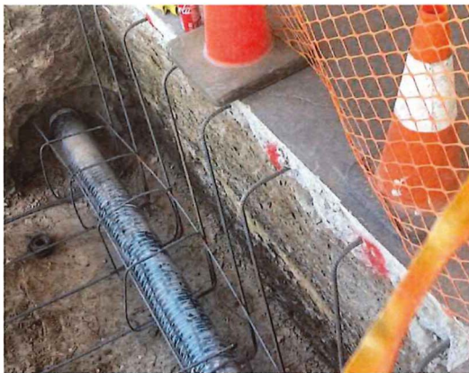
Waterline Change Order: Existing waterline was discovered to be in conflict with the original foundation design. New foundation was designed and approved by the city.
