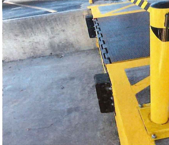
After: New leveler and bumpers installed for the dock
