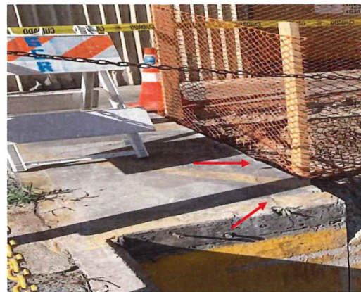
Slab Repair Change Order: Concrete replacement conducted on the existing damaged and cracked slab.
